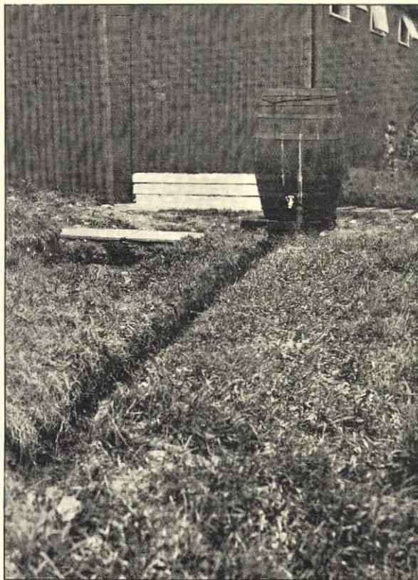
FIG. 3.—Barrel outside ablution shed showing channel for effluent and shallow pit on left into which sludge is emptied.
